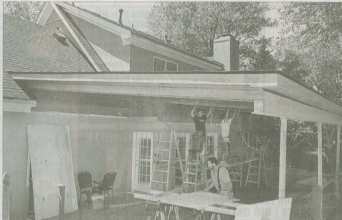
Employees of Atlanta Design & Build finish the ceiling over a porch during a remodeling project recently at a home in Roswell. “It’s not that a builder can’t do the work, but they think about the overall project much differently than we do,” says H. Dale Contant, president Atlanta Design & Build. Jason Getz jgetz@ajc.com
